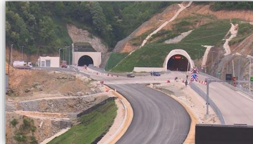
Tunel Tirana - Elbasan
